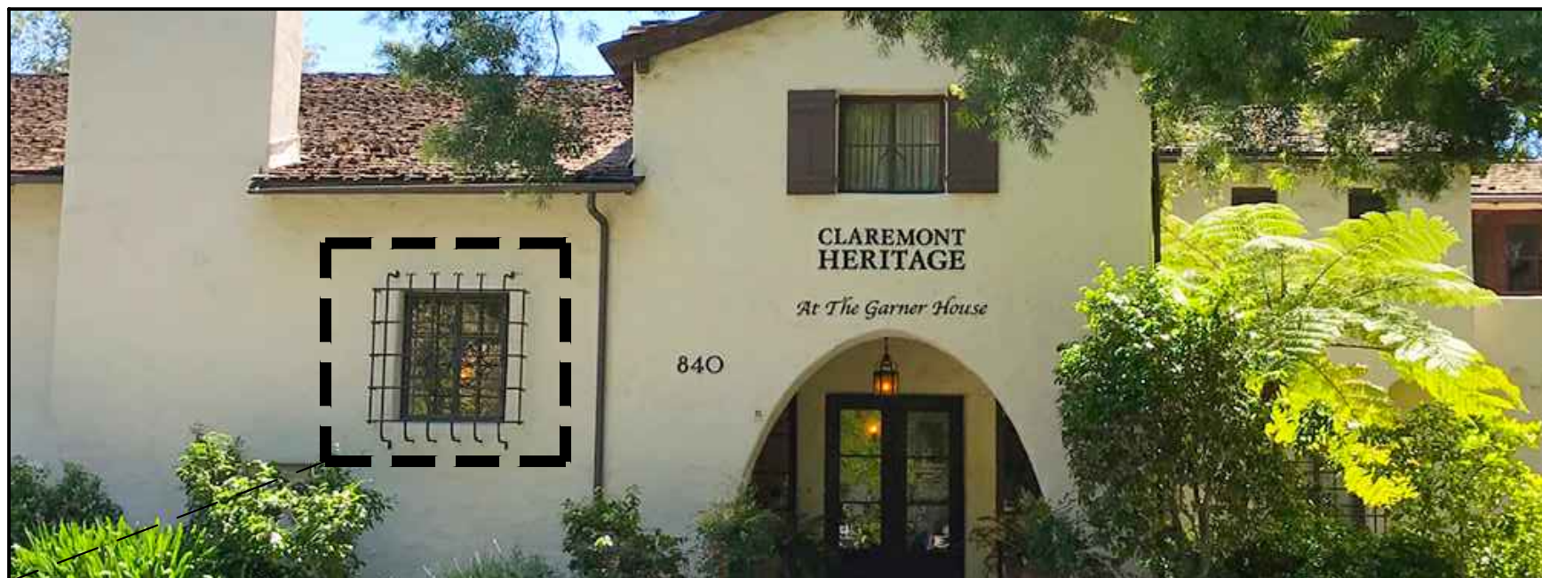
14. DECORATIVE METAL GRILLE WORK
