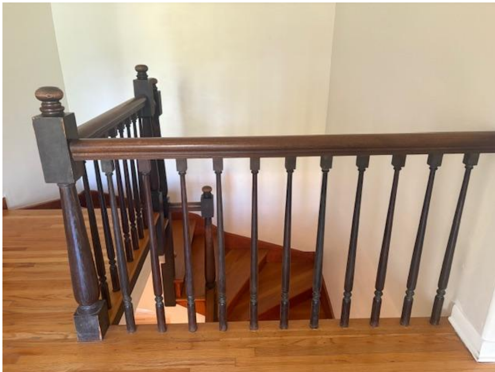
Historic staircase that does not meet current code for height of railing.
