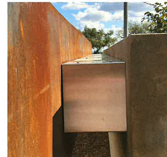
Aluminum box surrounds structural supports and electronics - matching existing RDSC signage
