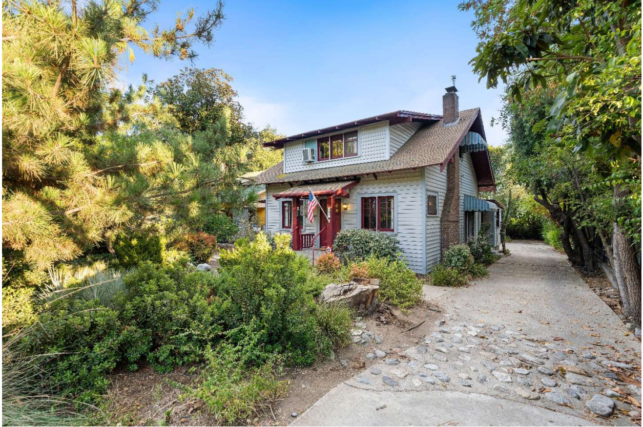
Front Façade, Looking Down the Driveway
