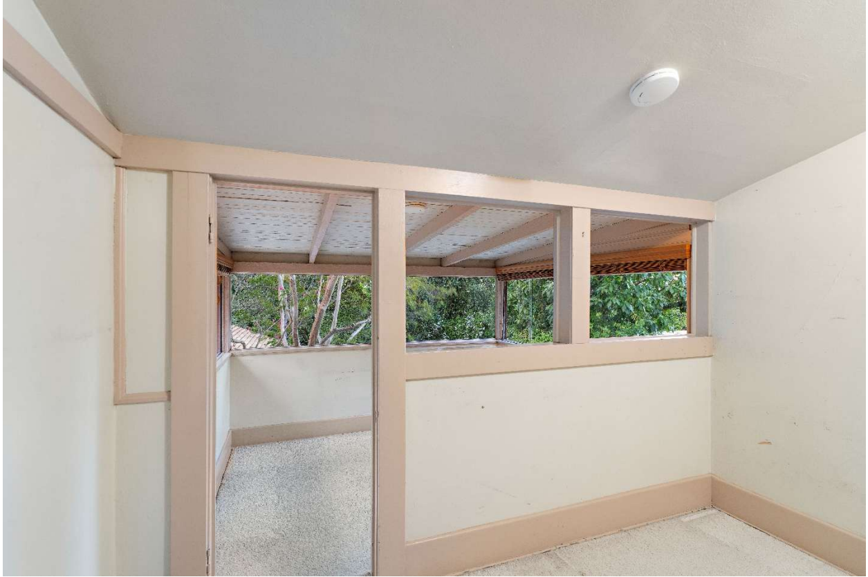
Second-Story “Look-Out” Rooms
