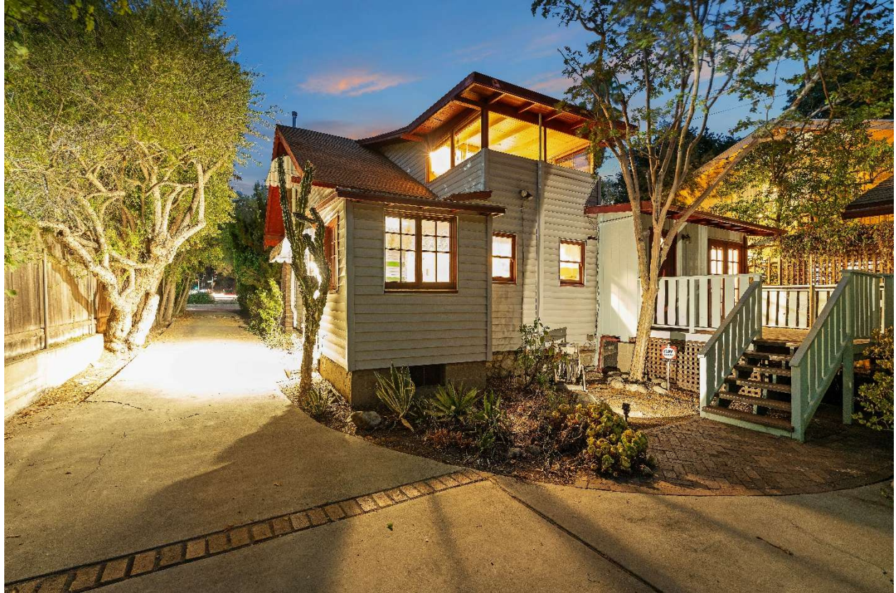
Rear Façade of Residence
