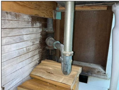
Corrosion is present at plumbing areas - this is a sign of slow leaking and should be further evaluated by a plumber. Master bathroom.
