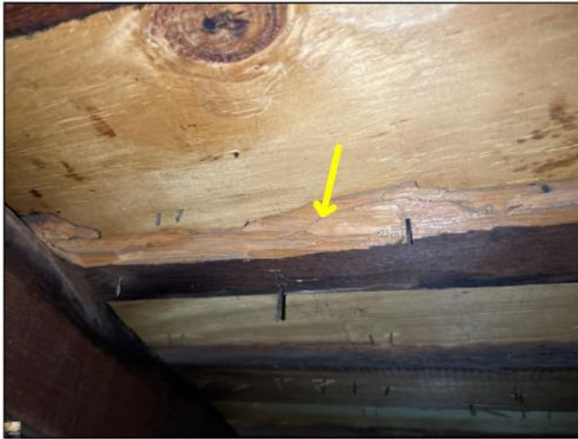
Deteriorated wood observed - consult termite report
