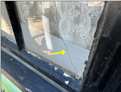
Cracked glass - needs to be serviced
