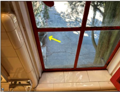
Cracked glass- needs to be serviced. Master bathroom.
