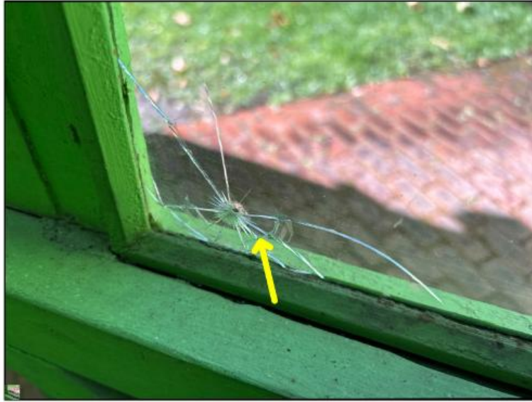
Cracked glass - needs to be serviced
