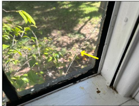
Cracked glass- needs to be serviced. Stairs bedroom.
