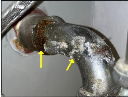
Corrosion is present at plumbing areas - this is a sign of slow leaking and should be further evaluated by a plumber. Master bathroom.
