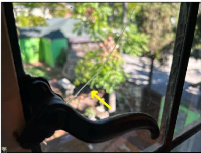
Cracked glass- needs to be serviced. Upstairs, Jack and Jill bathroom
