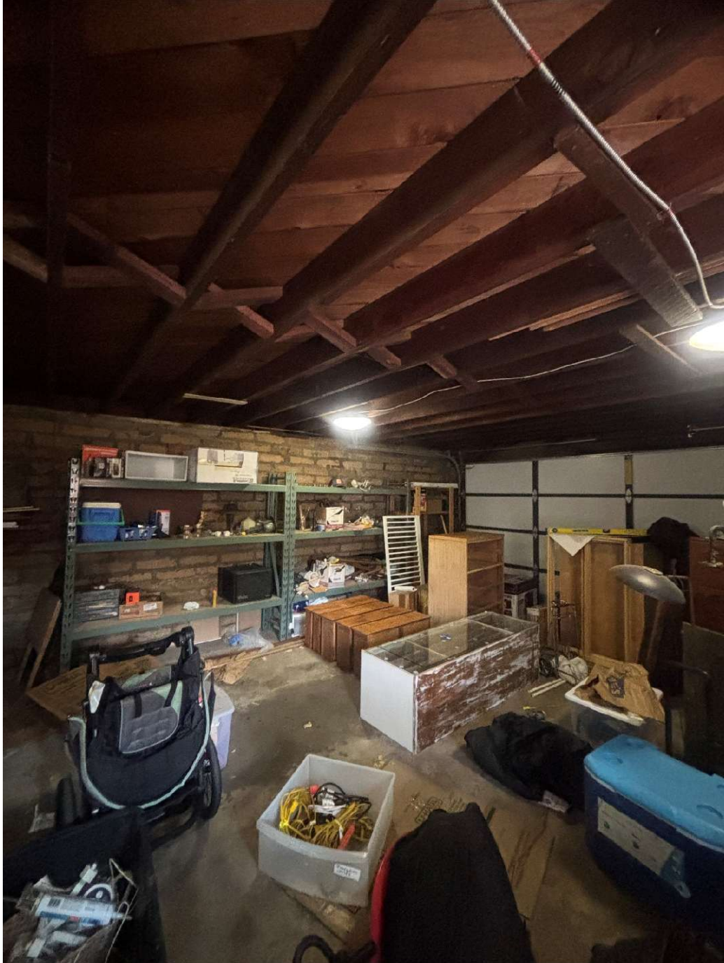
Detached Adobe Garage Interior
