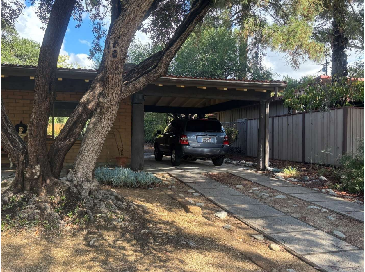
Attached Port Cochere and Driveway
