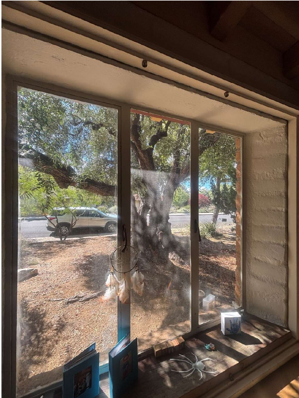
Casement Window in Bedroom
