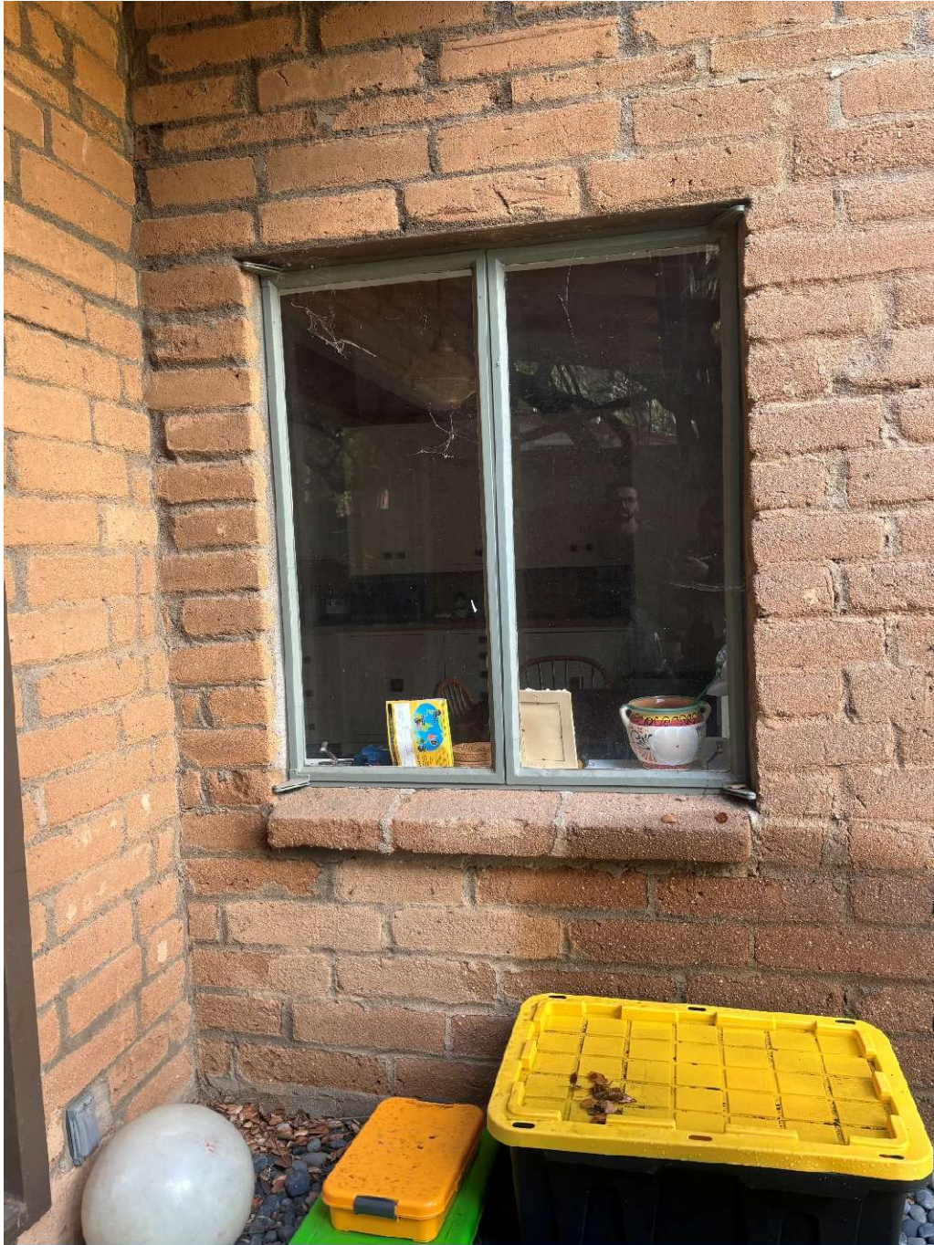
Exterior of Kitchen Window
