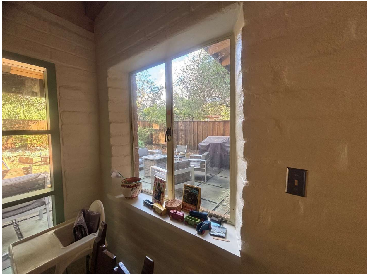
Casement Window in Kitchen
