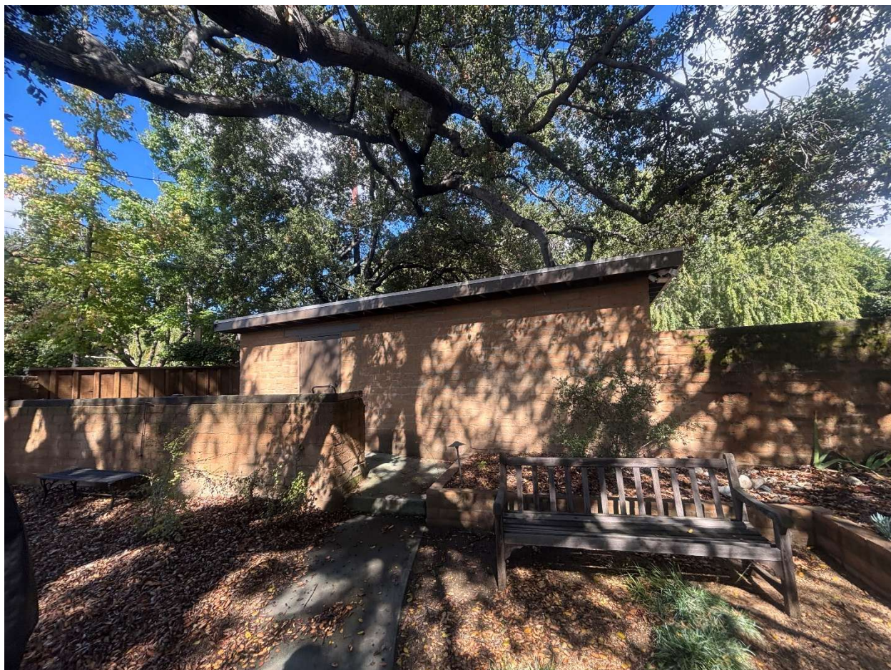
Detached Adobe Garage and Landscape Walls
