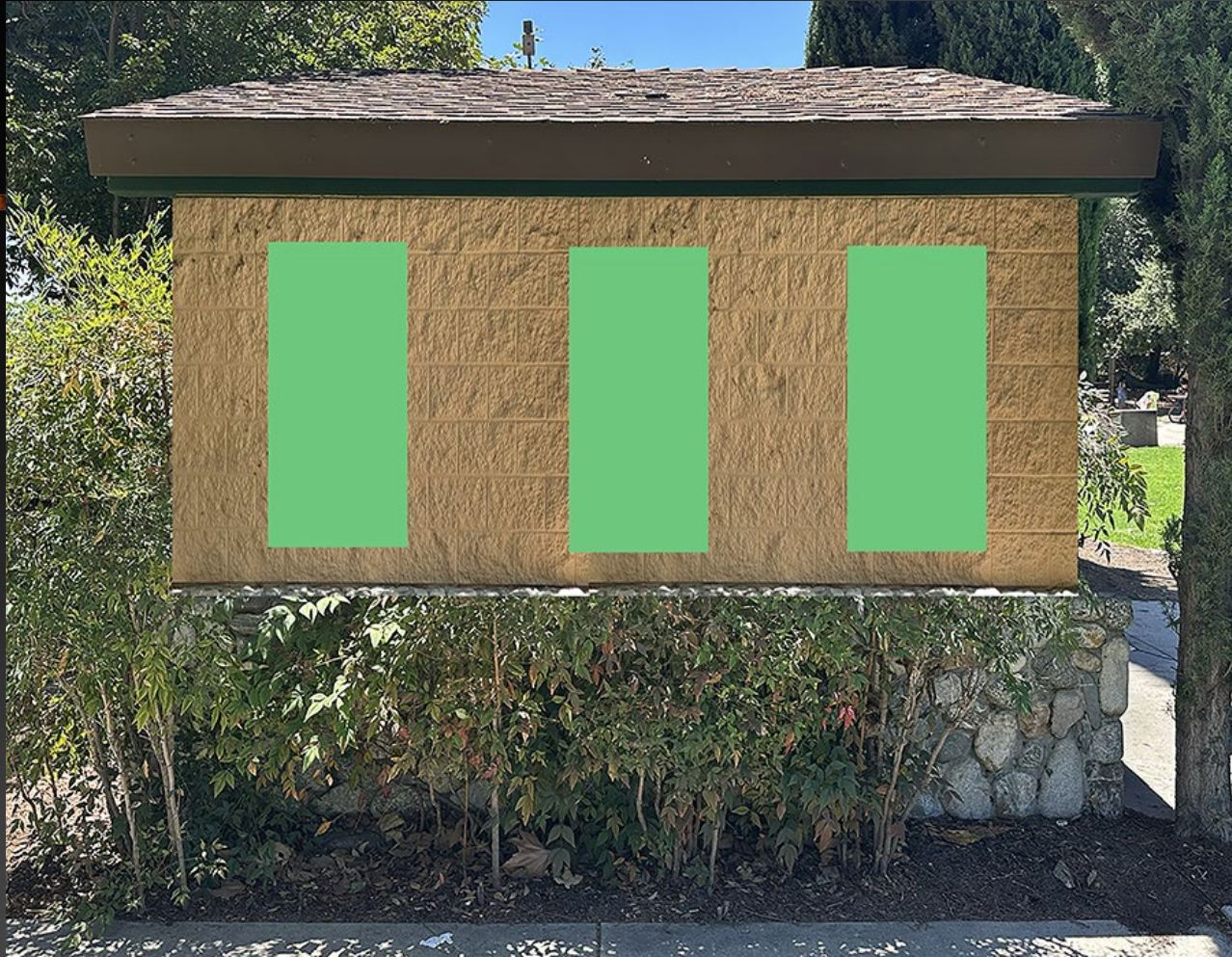
North Facing Wall
