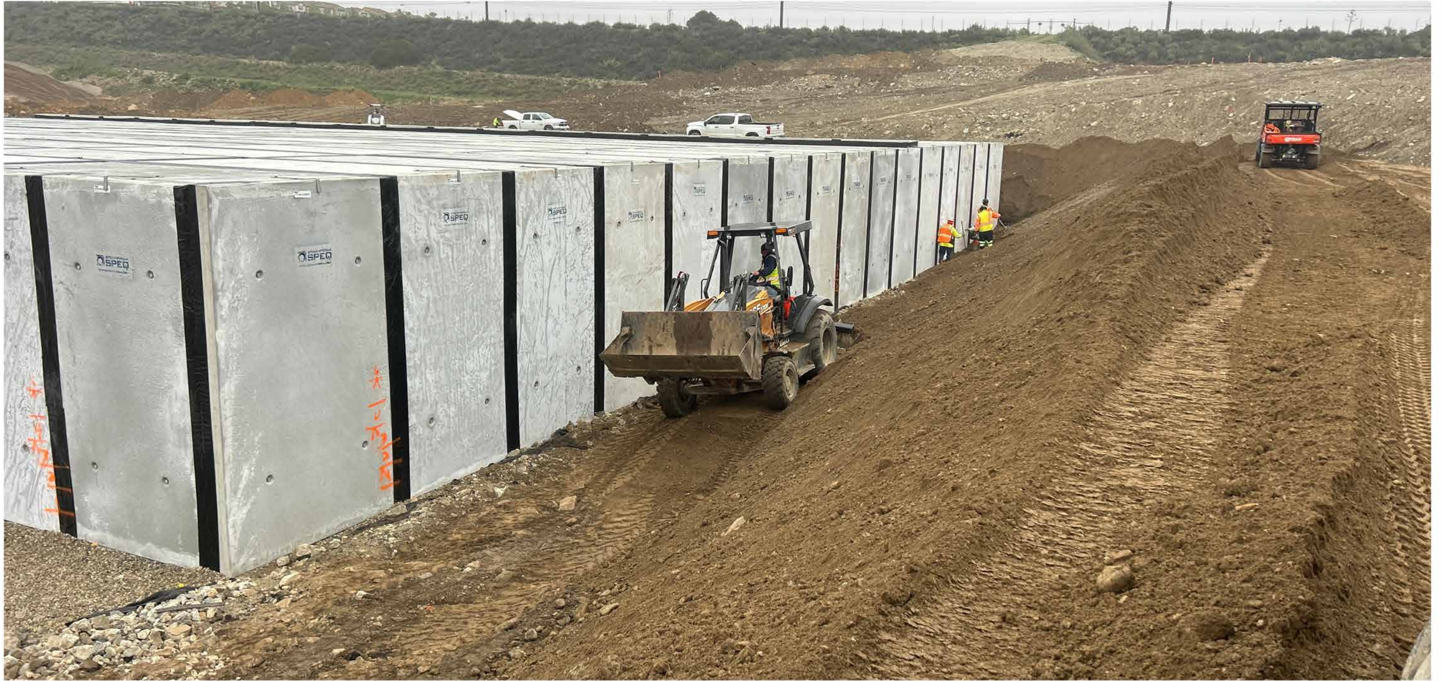
STORM WATER CHAMBER CONSTRUCTION
