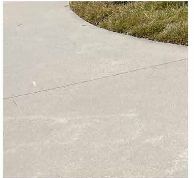
CONCRETE 'RETARDED' FINISH - CAMPUS STANDARD CONC-11
