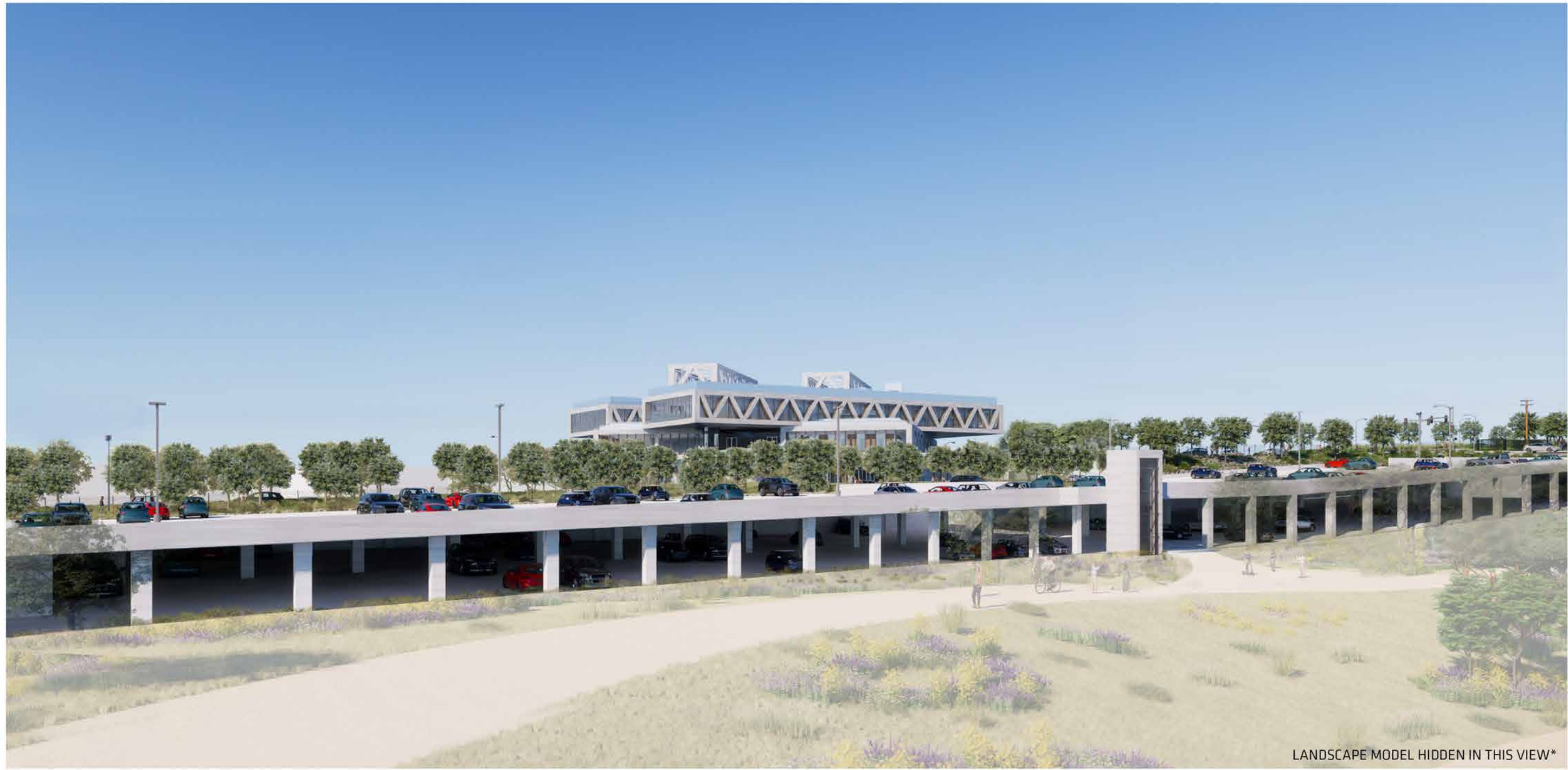
PARKING STRUCTURE EXTERIOR VIEW
