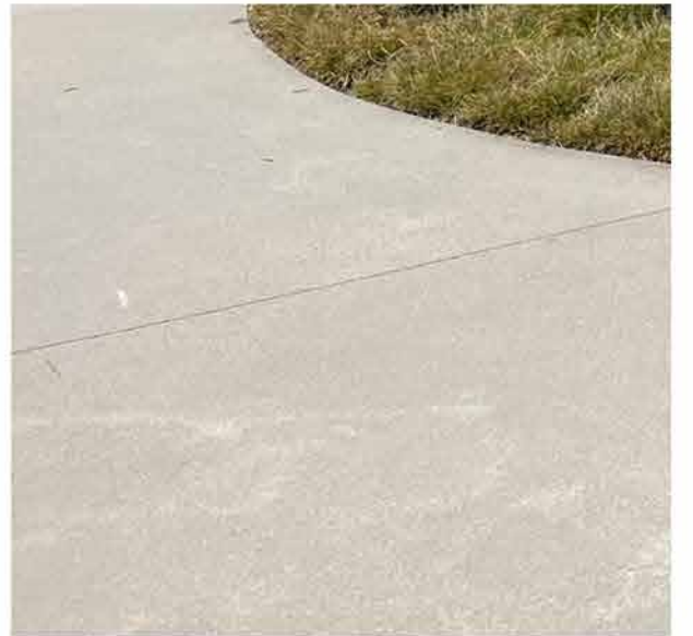
CONCRETE 'RETARDED' FINISH - CAMPUS STANDARD CONC-11
