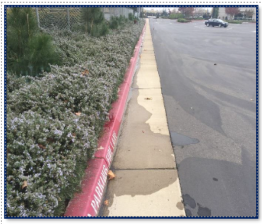
Photo 4: 1 Gallon Spill along a Curb (96 feet in length)
