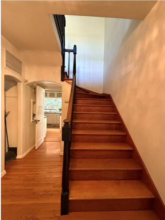
Historic staircase that does not meet current code for height of railing.
